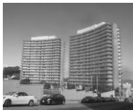
The Fontana Towers at Aquatic Park was an early loss for land-use battles. But the resulting planning war was won with passage of the waterfront 40-foot height limit---by the narrowest of margins.
